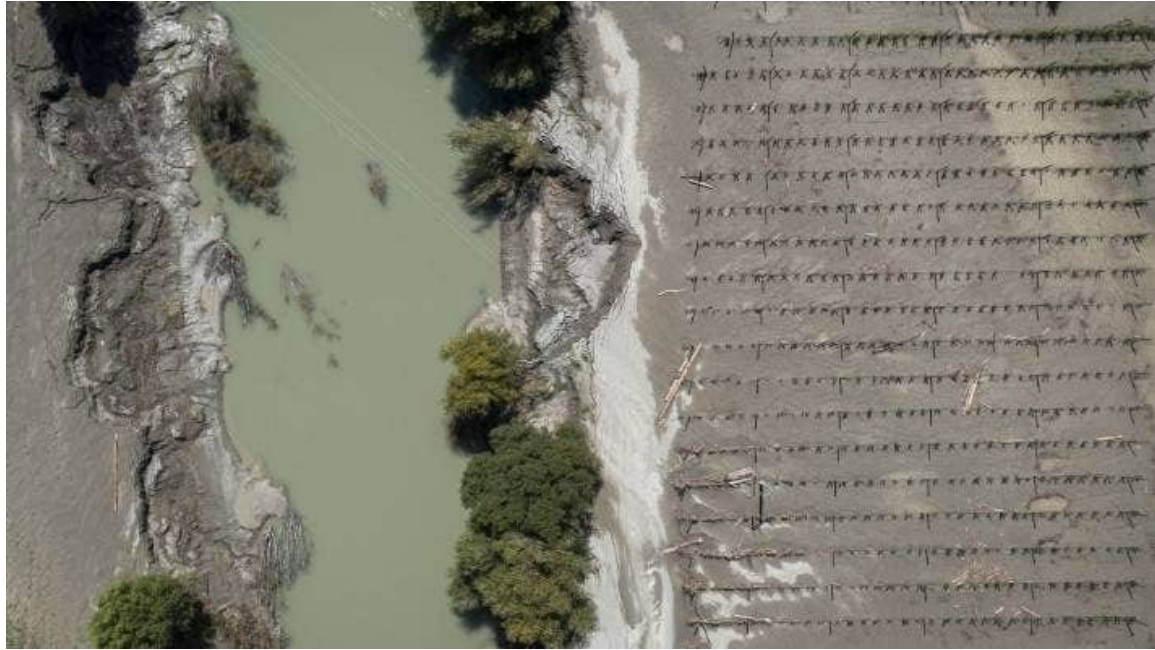
Damage to the Pine Valley Orchard which is on the banks of the Nuhaka River, between Gisborne and Wairoa.
